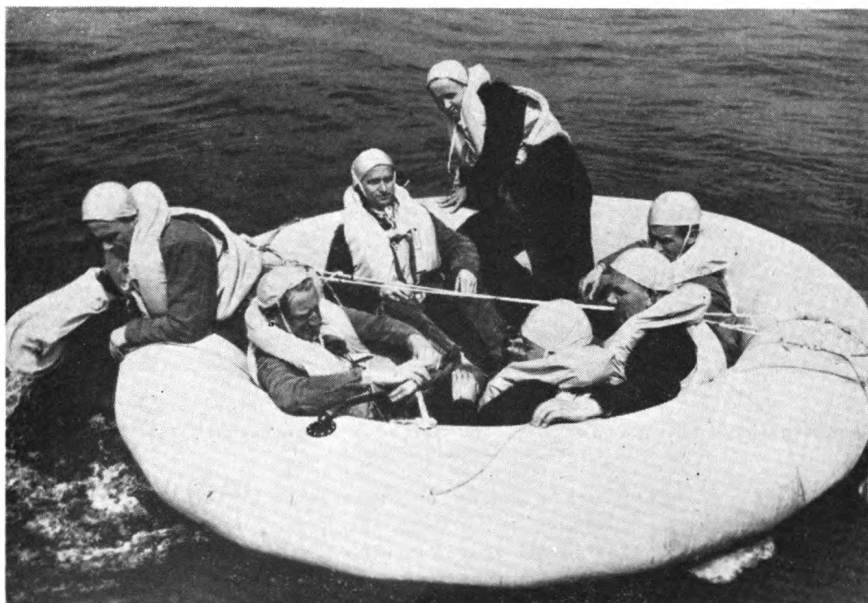
BRITISH LINDHOLME RESCUE DINGHY (One part of multiple unit assembly)
